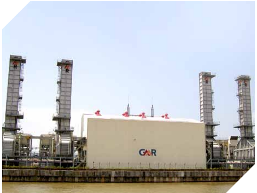
GMR ENERGY - 220 MW BARGE MOUNTED POWER PLANT
